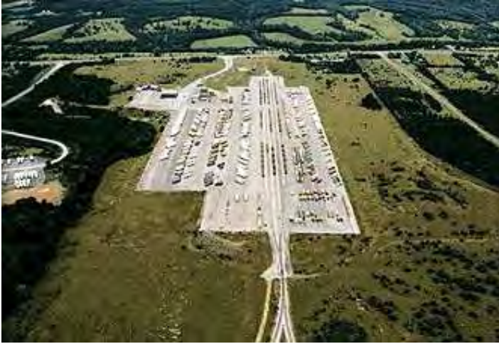
Figure 3.1 Aerial View of Virginia Inland Port
